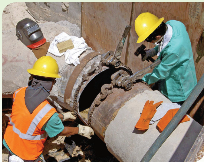
Crew from the BWS repairs a broken water main
