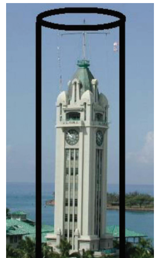
Aloha Tower will fit into each of the 20 Red Hill underground storage tanks. The Tanks were constructed inside Red Hill from 1940 to 1943.
