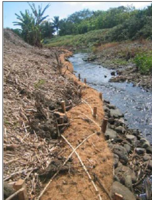
Example of "coir" erosion control technique.
