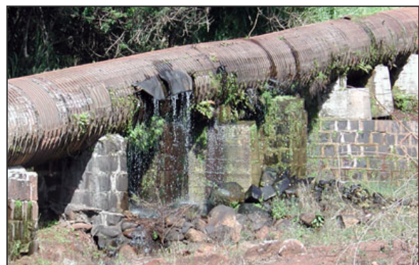
Siphons carrying Waiāhole Ditch water.
