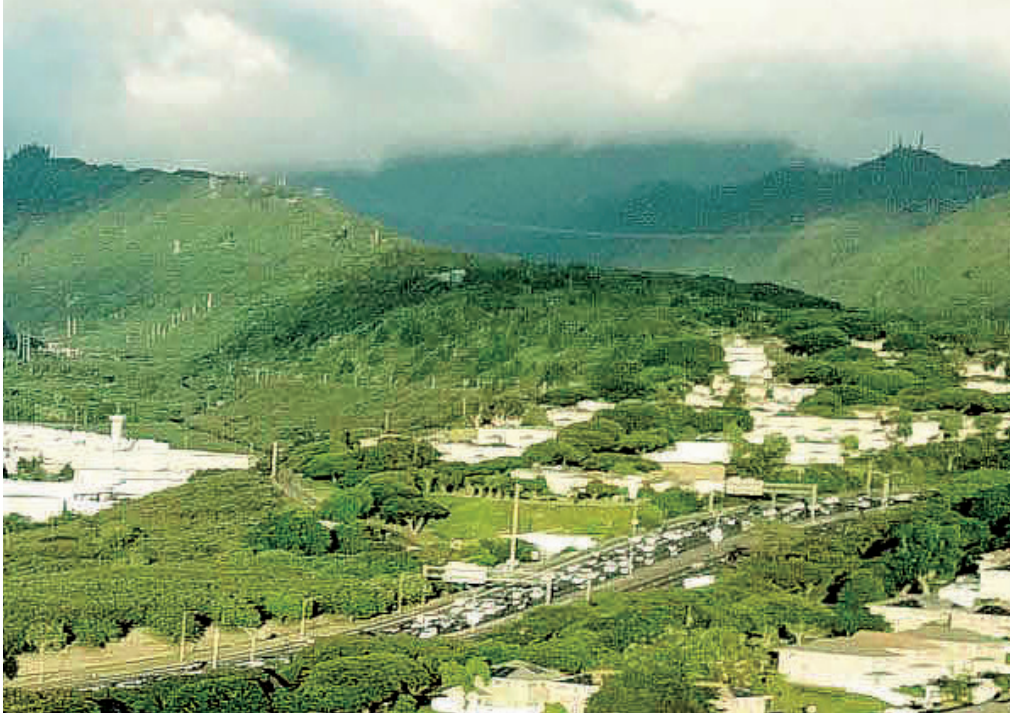
The H-201 Moanalua Freeway in the foreground, descends into Halawa Valley from Red Hill. The Red Hill fuel tanks are buried inside the hillside, just 100 feet above Oahu's pure water source.
