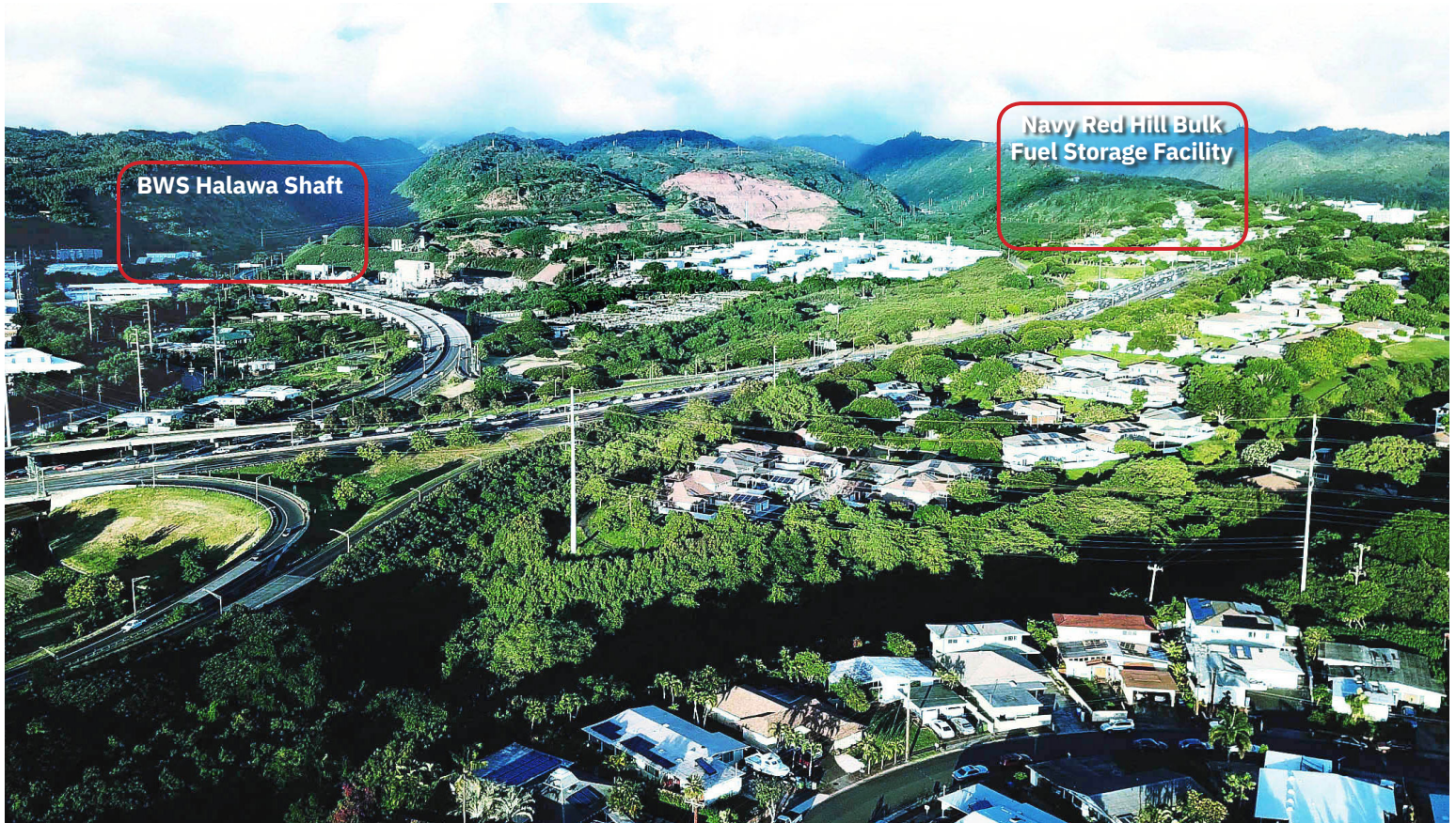
The U.S. Navy Red Hill Bulk Fuel Storage Facility can be seen above on the right, while the BWS Halawa Shaft can be seen on the left.
