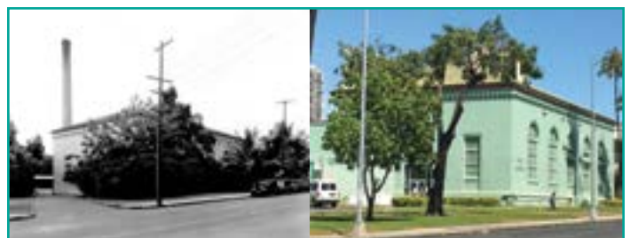
Beretania Pumping Station Then: 1935 and Now: 2016
