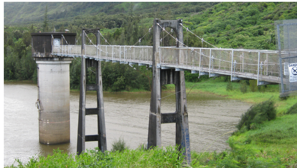
Nuuanu Reservoir No. 4 features a tower through which water drains from the reservoir pool.
