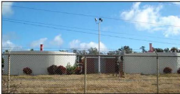
Waimānalo WWTP facility
