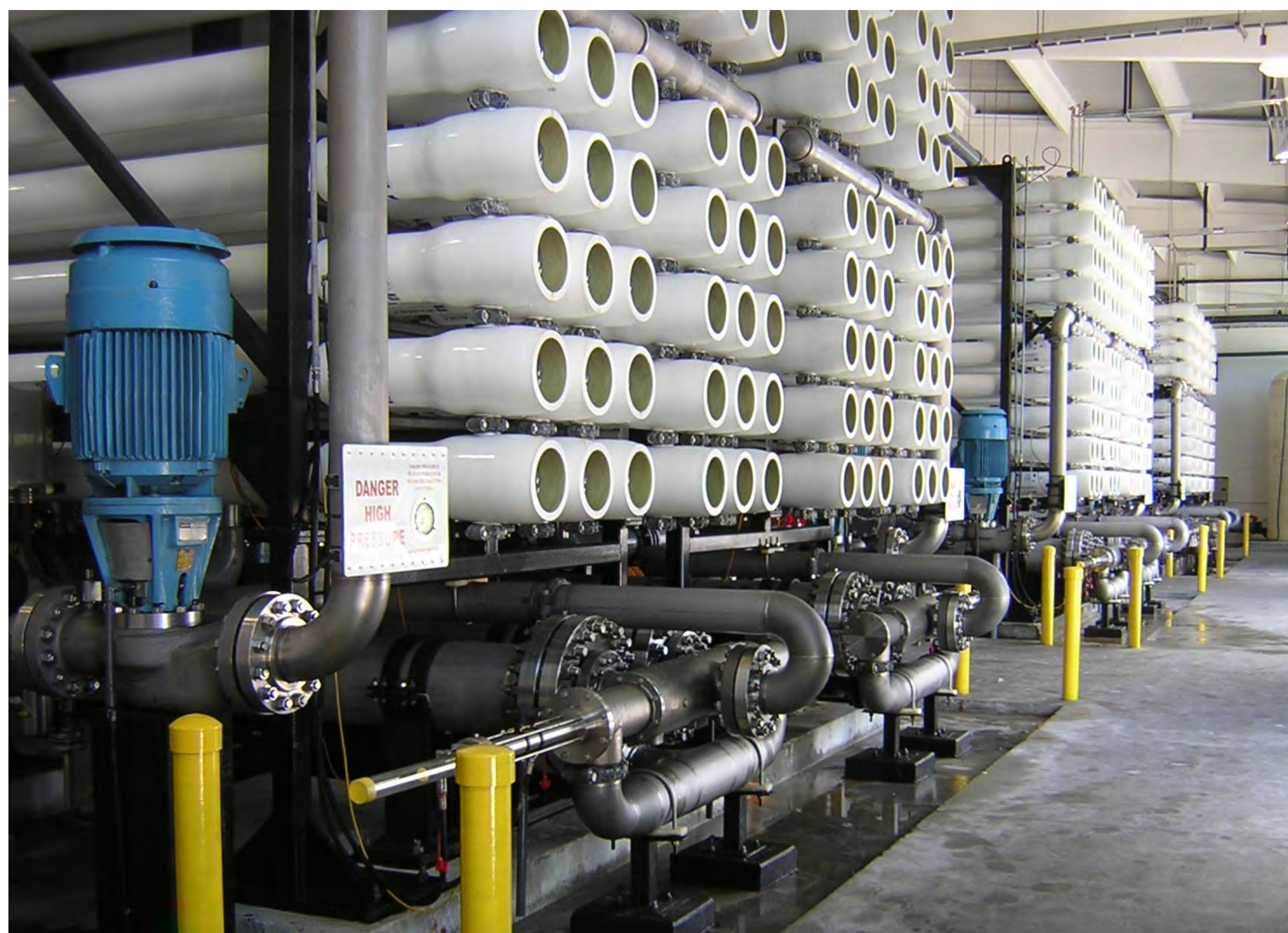
Typical Kalaeloa Desalco Seawater Reverse Osmosis Facility designed, built and operated by Kalaeloa Desalco.
