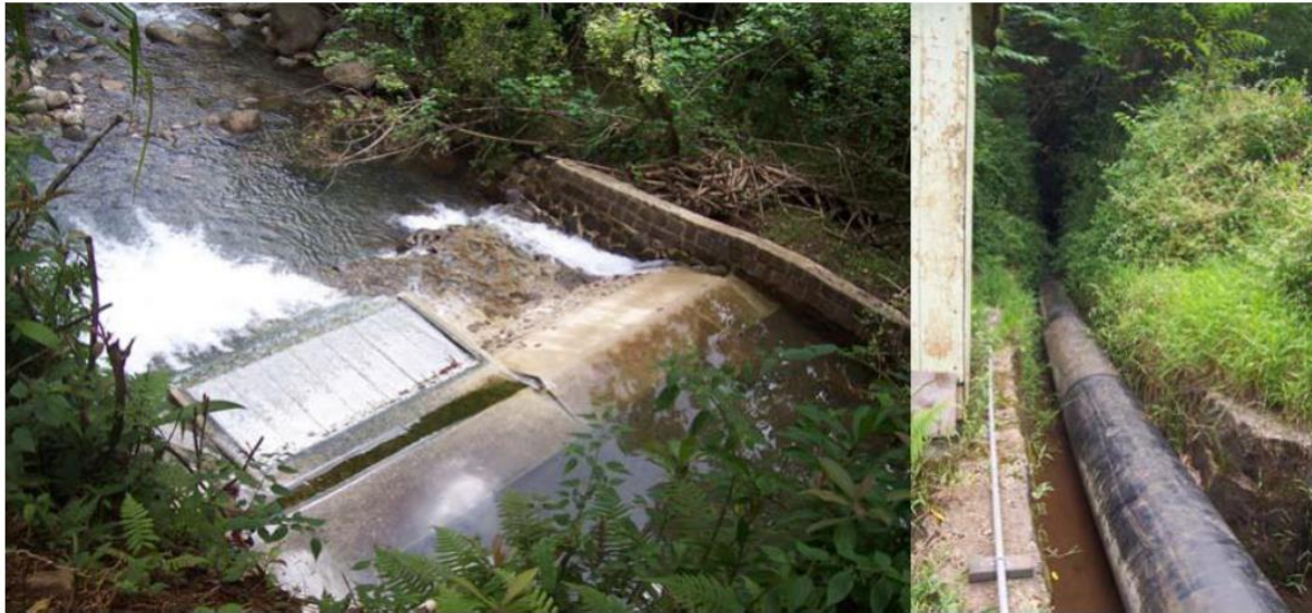
Figure 1-8: Punalu'u Stream Diversion and Piped Ditch
