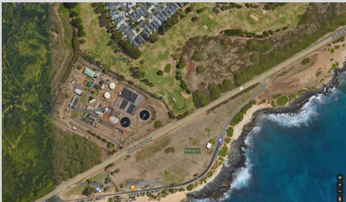
Image: Aerial View of the East Honolulu WWTP (Credit: Google Earth).
