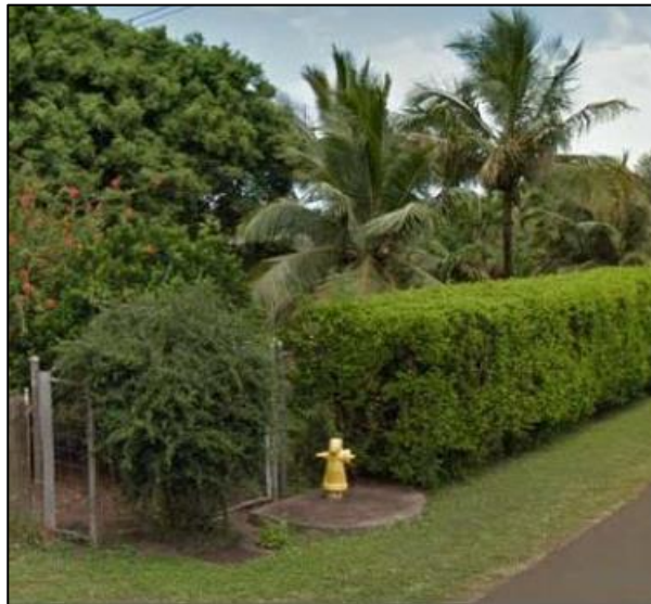
City fire hydrant that is more than one mile from nearest Mokulē'ia residence
