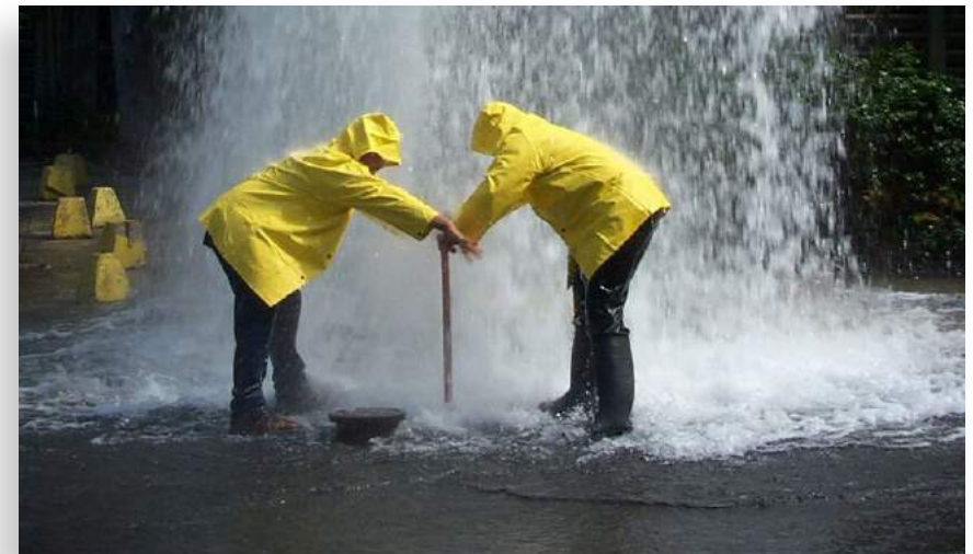
Targeted pipe replacement prioritized based on highest risk can significantly reduce main break rates and increase pipe replacement efficiency.
